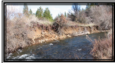
This severely eroded bank is a prime candidate for restoration
